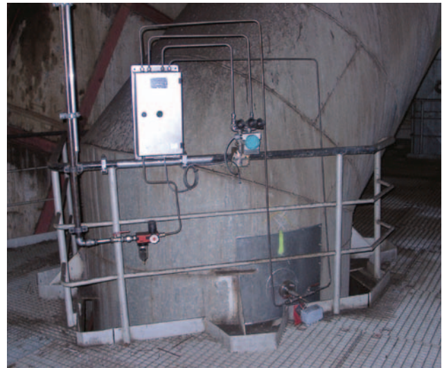
DF25 with LSP air purging system for combustion gas with high particulate content after air preheating.
